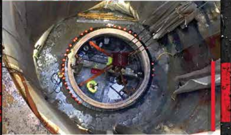
160 FEET DEEP (48.8 METER) UTILITY ACCESS 14 FEET (4.3 METER) DIAMETER PRECAST MANHOLE
