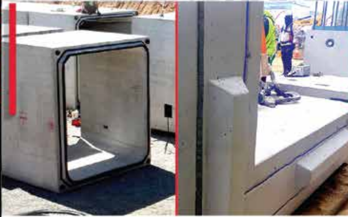
1 MILLION GALLON WATERTIGHT STORMWATER DETENTION SYSTEM
