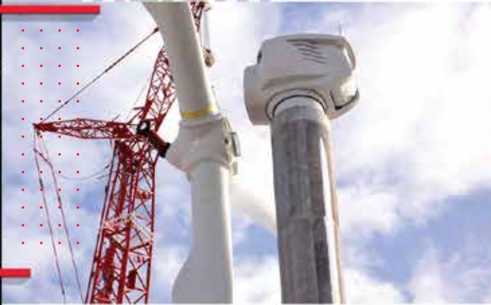
100 METER TALL (328 FEET) PRECAST WIND TURBINE TOWER
