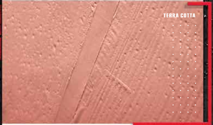
COLOR MATCHED WATERPROOF COATING & ELASTOMERIC JOINT SEALANT APPLIED TO ARCHITECTURAL CONCRETE JOINT
